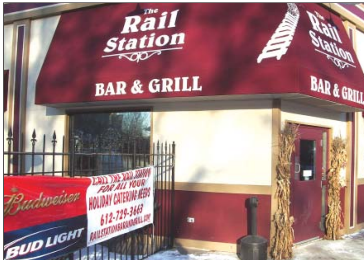
The Rail Station Bar & Grill moved into the old Jimmy's Steakhouse, a windowless bar, in July 2003. Former patrons of Jimmy's wouldn't recognize it now. The Rail Station put in many large windows, completely redid the exterior, installed a new patio and awnings, and just opened a "smoking car" beside the building.
